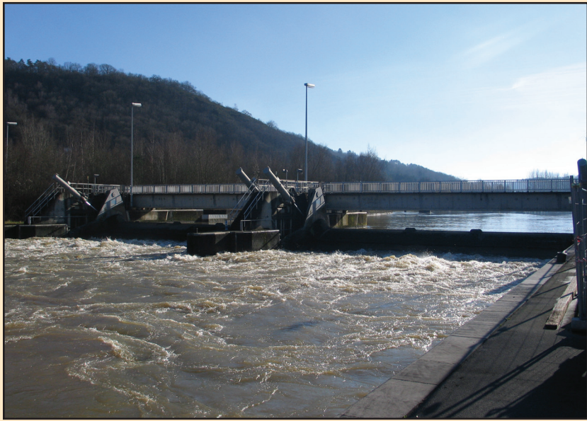
Figure 5. On the Meuse River, gates move according to feedback laws constructed by Jean-Michel Coron and his colleagues. Photo credit: Jean-Michel Coron.
